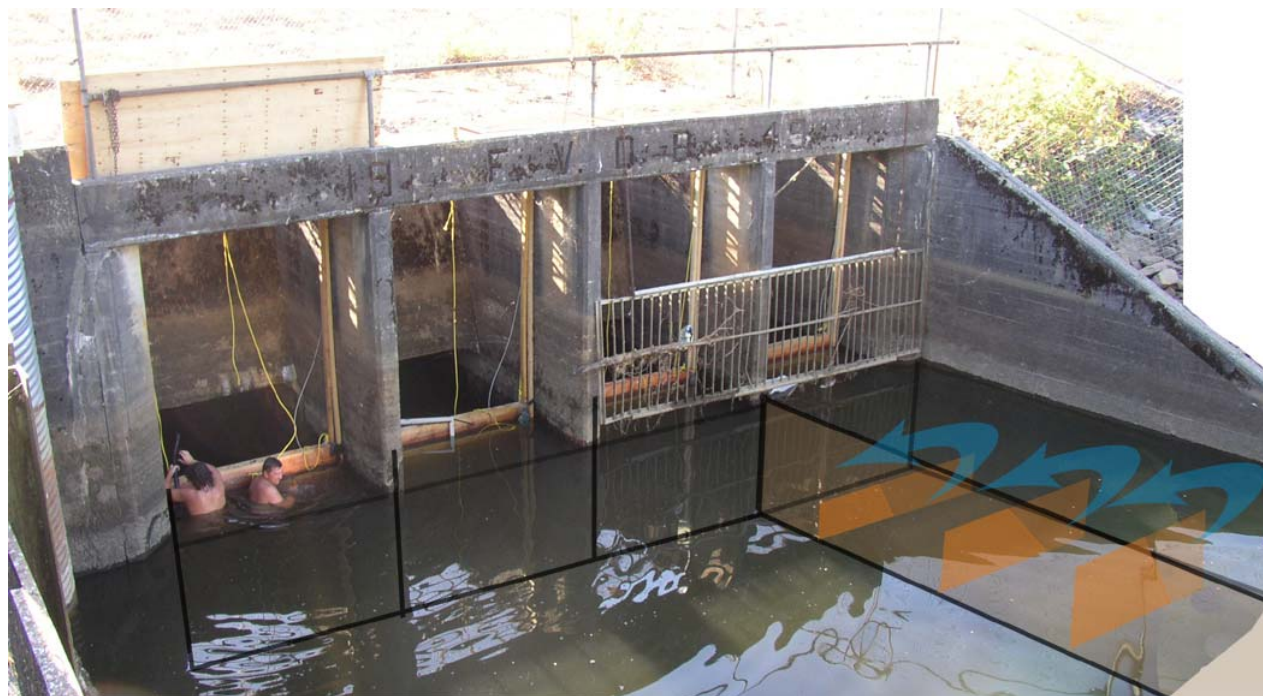
Proposed concept - fish access weirs on north flood box (photo from 2003 installation)
